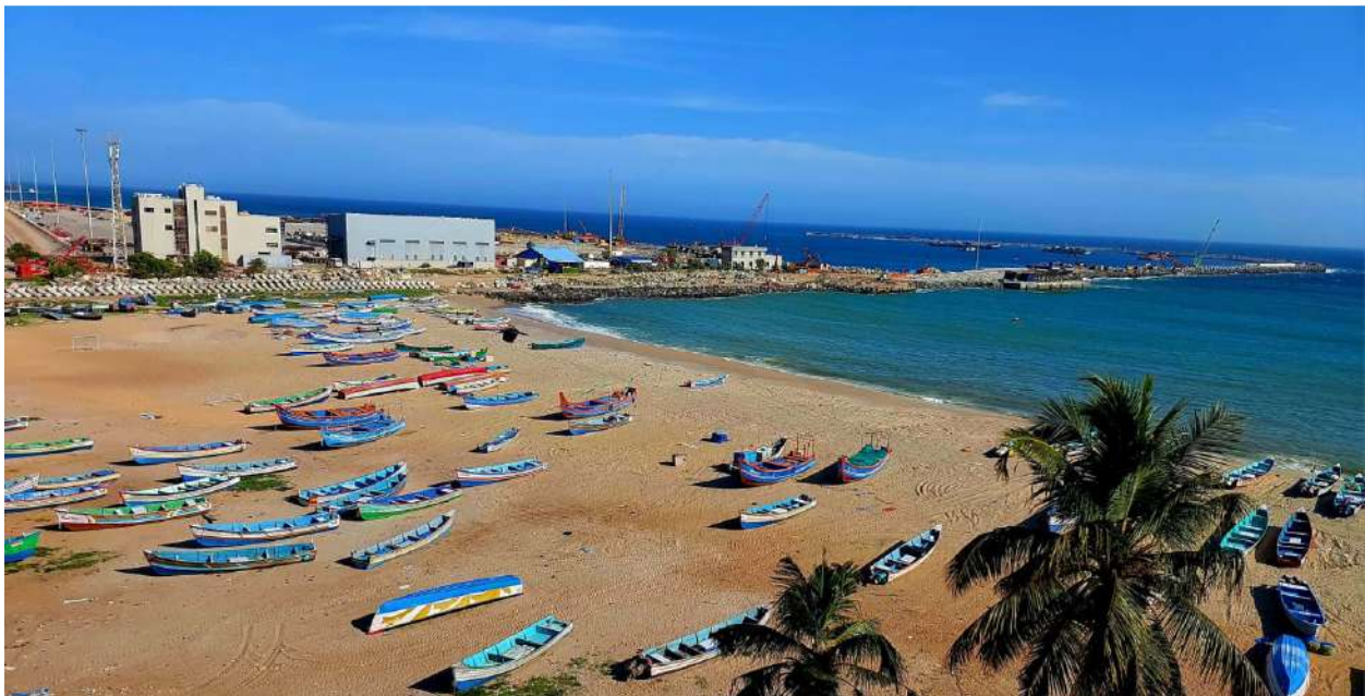
Fig 5.22: Substantial beach building observed at Valiya kadapuram adjoining to and between the harbour mouth and the port breakwater under construction Credit: Probir Banerjee
