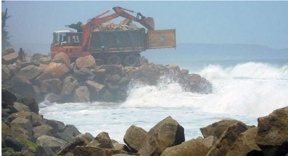
Groyne construction in progress in Valiyathura.
