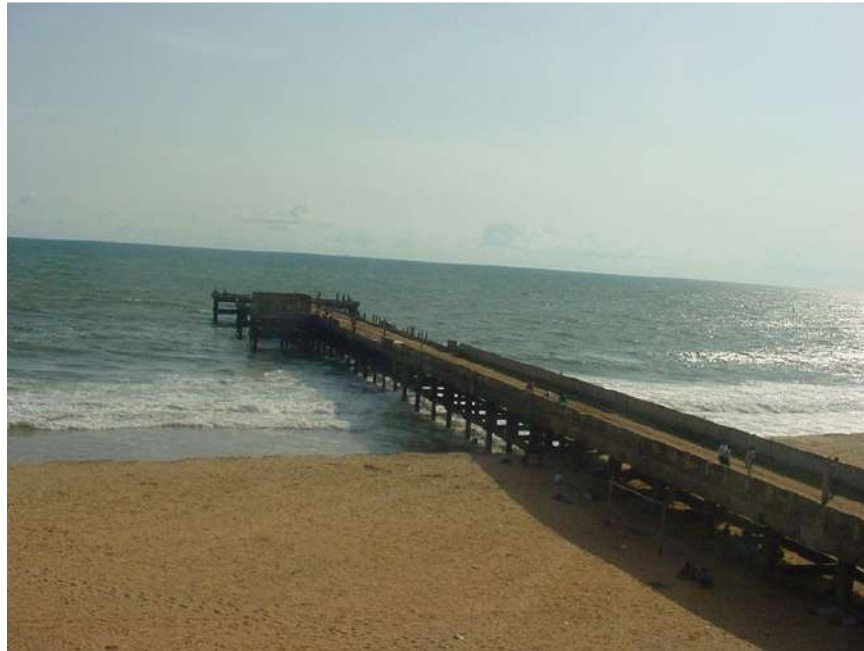
Fig. 5.15. Wide beach and the pier at Valiyathura prior to commencement of port construction
