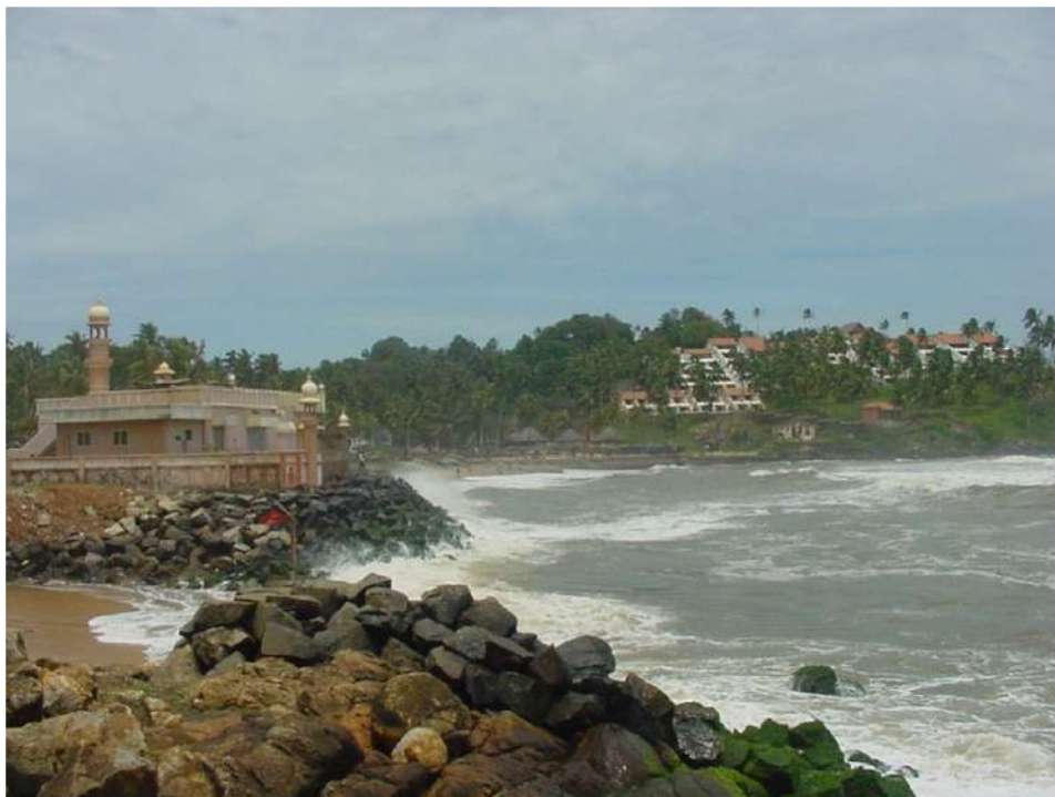
Fig. 5.7. Kovalam - Once there was a very wide beach seaward of the building (even during monsoon season) which was built (in 1984) landward of the monsoonal berm crest – best example of what happens with interventions on beach processes (Credit: K V Thomas)
