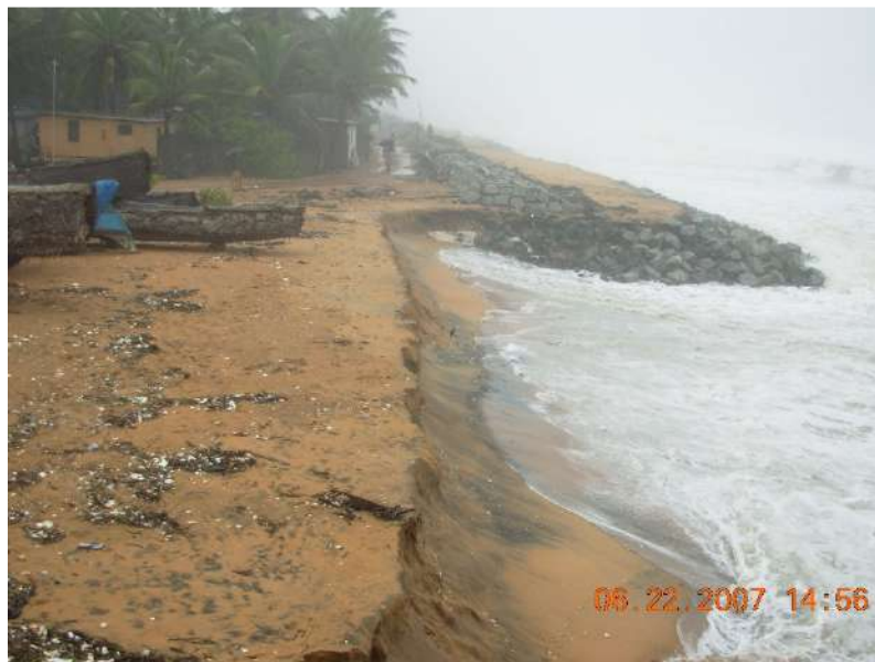
Fig. 5.9a. Low seawall with beach on its seaward side even during monsoon at Valiyathura (Photo: June 2007)
