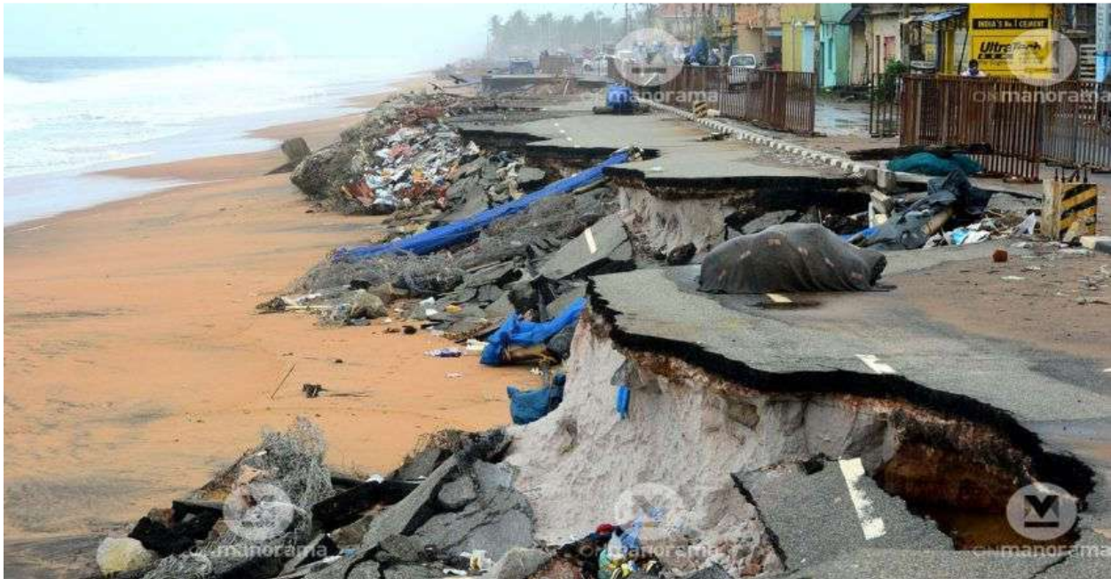
Fig 8.3: Shangumukham Beach Road to the Trivandrum International Airport destroyed by the waves. File photo: Manorama
