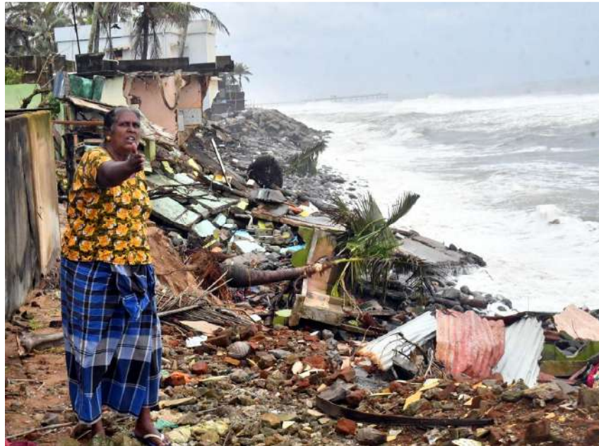
Fig 7.2: Shangumukham Beach Road in 2021 impacted by coastal erosion north of the VIS (Valiyathura Pier in the background)
