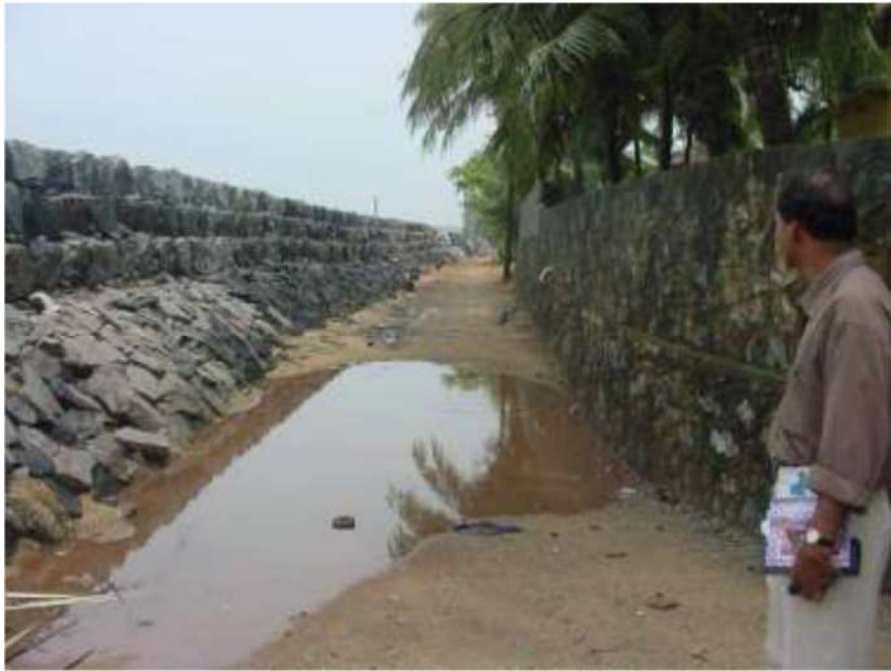
Fig 10.3 Between seawall and Compound Wall! Credit: KV Thomas
