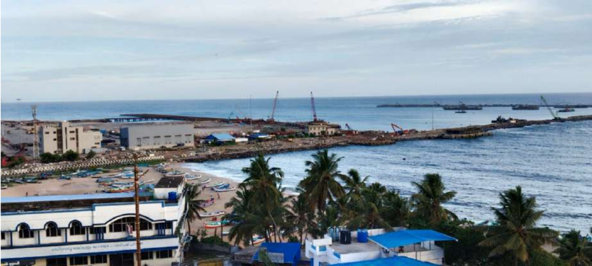
Fig 11.1: VIS Breakwater as on June 3, 2023
