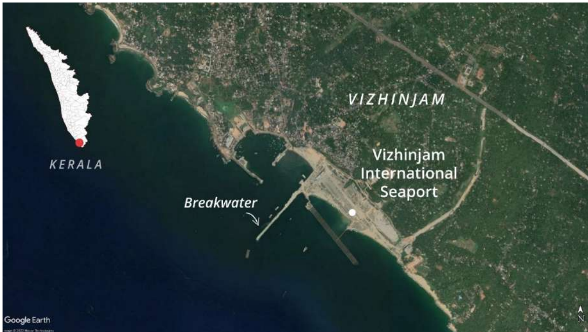
Fig. 5.10. The site of Vizhinjam International Seaport. Breakwater of about 1 km protrudes beyond the headlands. Base map from Google Earth; Breakwater further turns south and proceeds parallel to the coast for another 2.18 km in the first phase (under construction)
